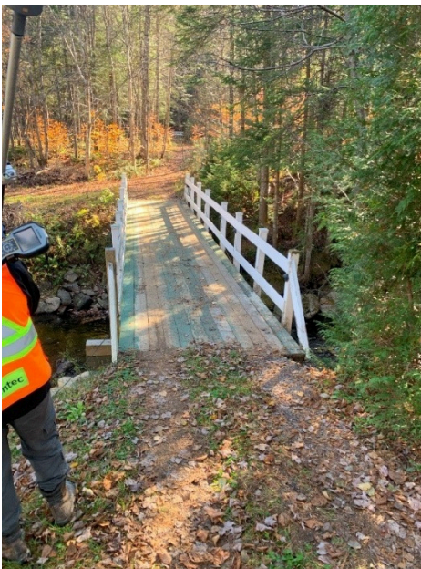
Figure 7-3 : Pont acier-bois PK 2+270 m
