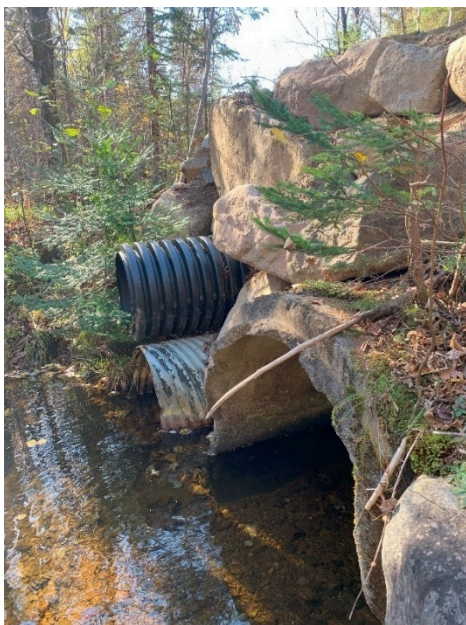
Figure 7-7 : Amont ponceaux PK 2+550
