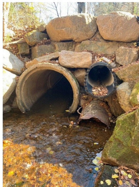
Figure 7-8 : Aval ponceaux PK 2+550
